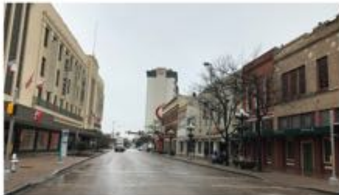
ALAMO PLAZA - EXISTING CONDITIONS
