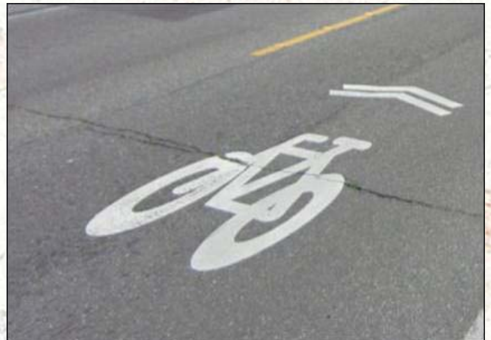
“Sharrow” Pavement Markings
